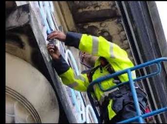
Technician from Neon Circus fabrication studio repairs failed units Photo: Neon Circus
